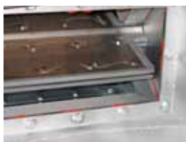
(Above) Interior view of Air Valves with silicon seal (red)
