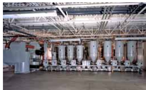
Above (Top): Side View of Large DHD Dryer, Floor Mounted, for Central Drying Configuration.
